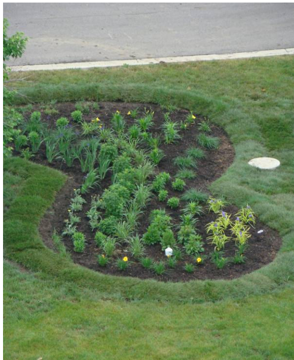
The planting plan incorporates a diversity of perennial plantings to help filter urban runoff.
