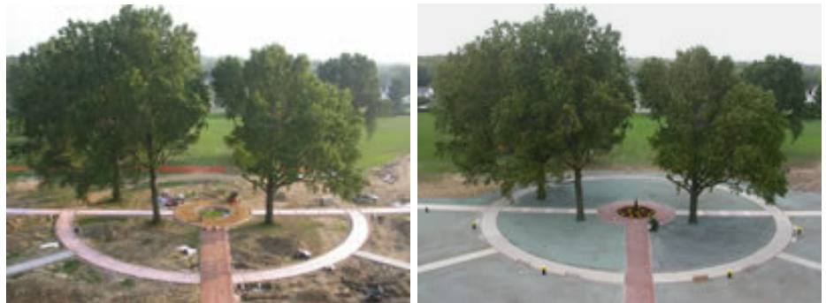
Construction photos of the Quinlivan Circle
