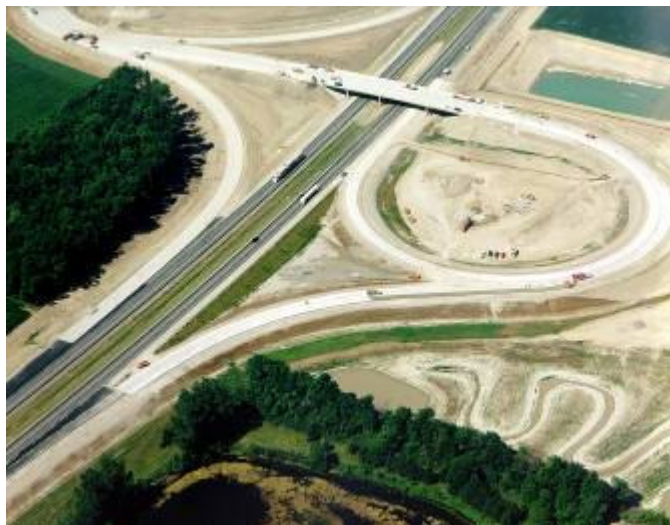
The constructed wetland serves wetland mitigation, earth borrow, and stormwater treatment purposes.
