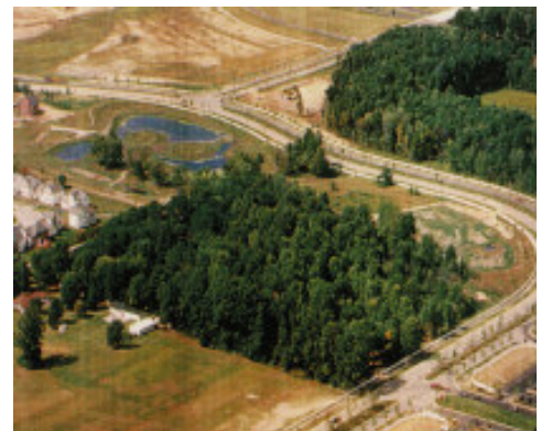
More than 13 acres of forested, emergent and seasonally inundated wetlands were constructed.
